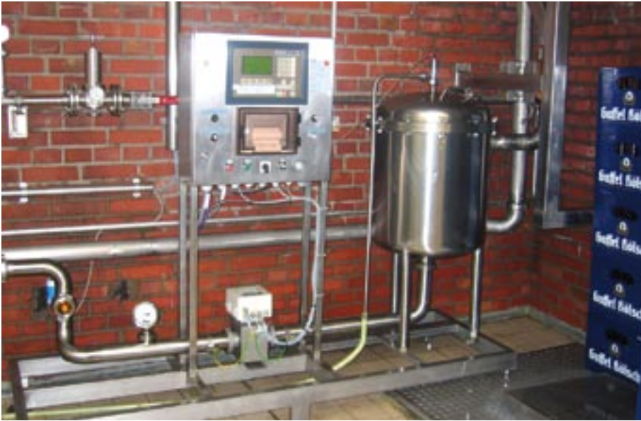
Figure 2: Officially approved beer delivery equipment gas separator and printer
