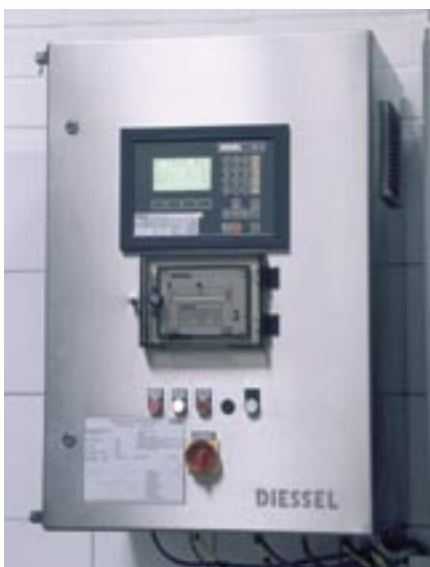
Figure 9: ZEVODAT operating and display unit
